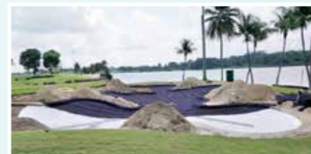
Overlaying of new sand mats for better drainage.
