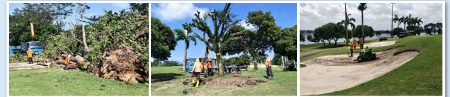
Restoration works in progress.
