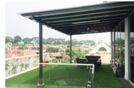
Aluminium Composite Panel with Metal Structure
