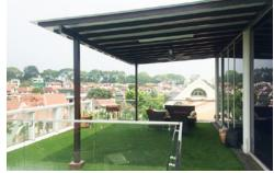
Aluminium Composite Panel with Metal Structure
